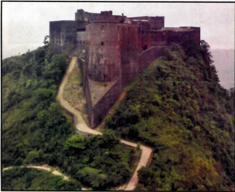
The Citadelle Laferriere, Built in 1820 The largest fort in Western Hemisphere
